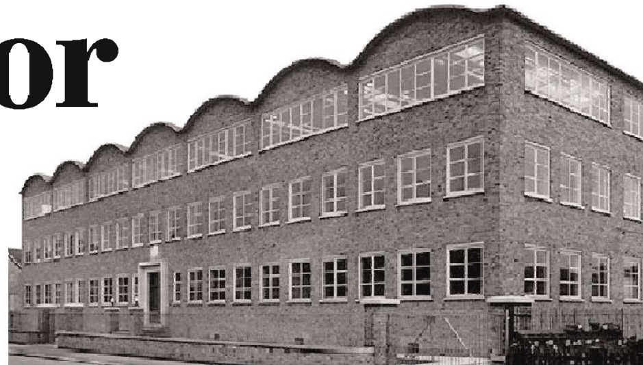
REJUVENATION: The Factory is part of major development on the brownfield site around the Riverside area in Norwich.
